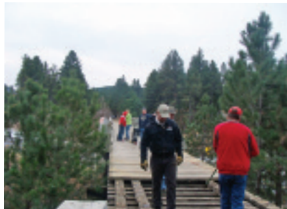
South Dakota union members rebuild a hiking trail bridge.
